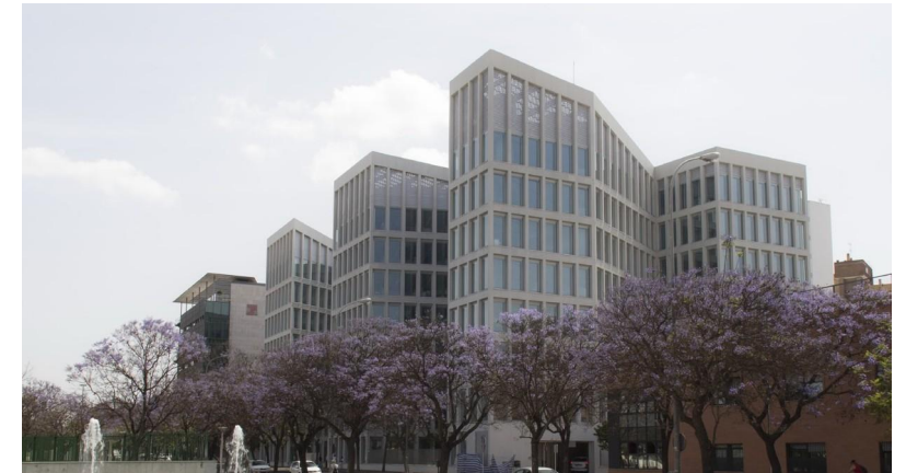
Headquarters in Seville
